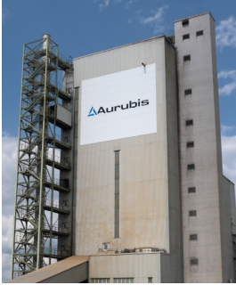
South view of the Kayser Recycling System
